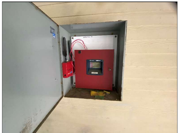
84. Central fire alarm panel in breezeway
