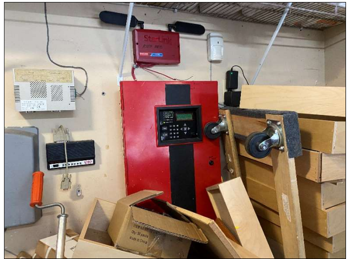
82. Central fire alarm panel in maintenance shop
