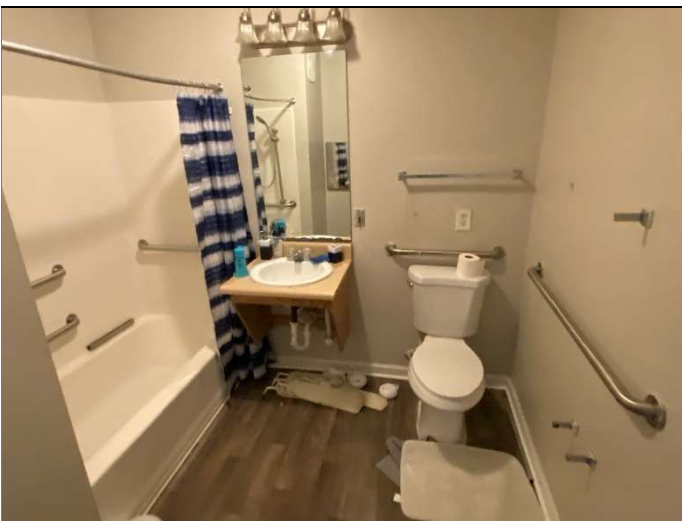
125. Type A/UFAS accessible dwelling bathroom; note call station
