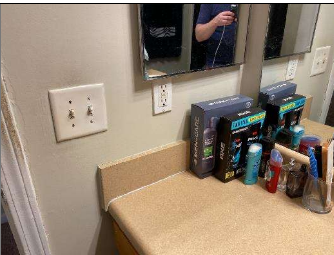
77. GFCI receptacle protection bathroom outlets
