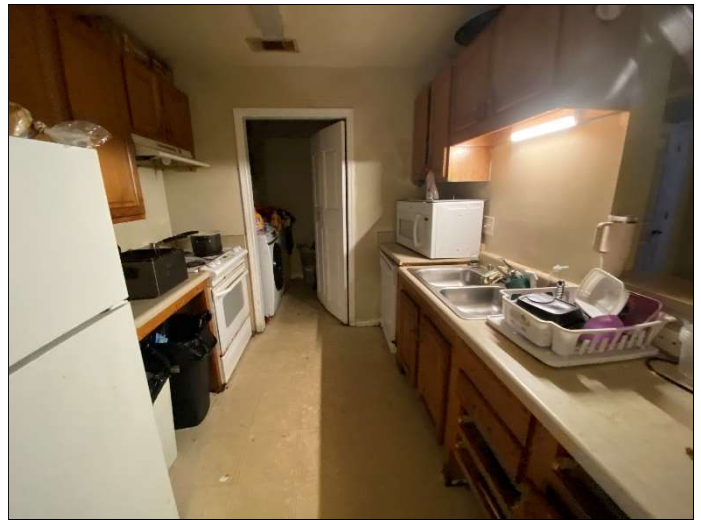
124. Type A/UFAS accessible dwelling kitchen without a range-oven clear floor space
