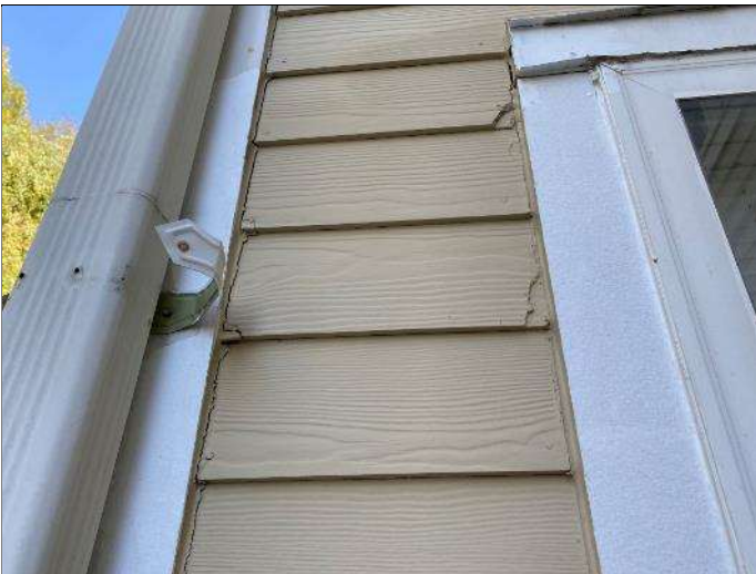
51. Deteriorated sealants and fasteners
