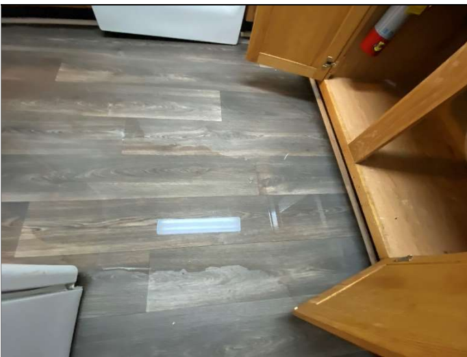
59. Water standing in floor from leak in C308.
