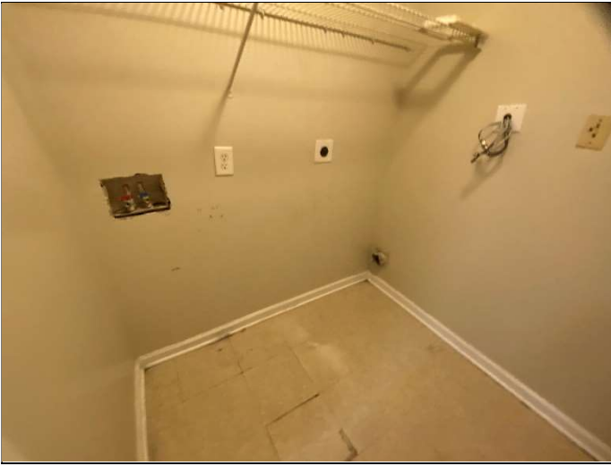
79. No GFCI protection at a laundry room washer outlet
