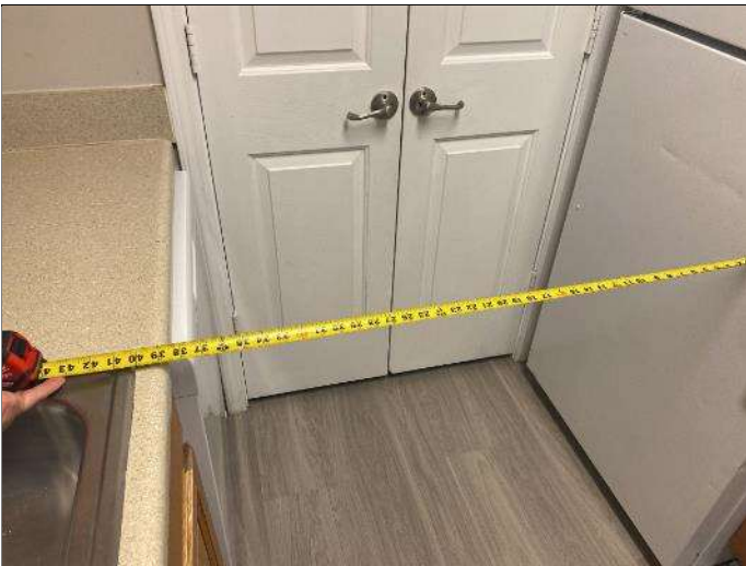
117. 2 BR kitchen galleys less than 40" between fridge and dishwasher
