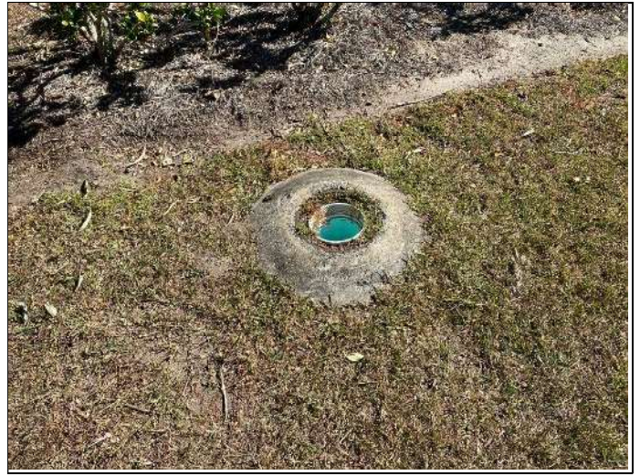
44. Sanitary sewer cleanout missing a cap
