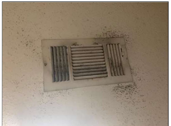
72. Dust accumulation indicative of dirty filters/ducts
