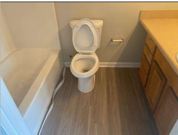
119. 3 BR master bathroom without a lavatory clear floor space
