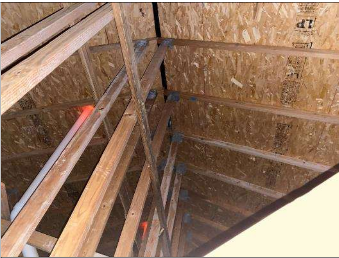
45. Roof trusses and OSB decking
