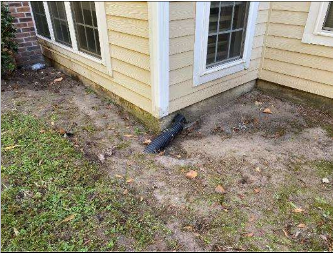
61. Building G downspout disconnected from discharge
