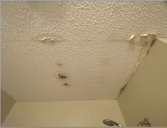
109. Aged water staining and growth on a ceiling. Unit 201.
