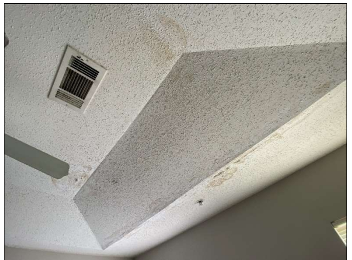
108. Roof leak in Unit 304
