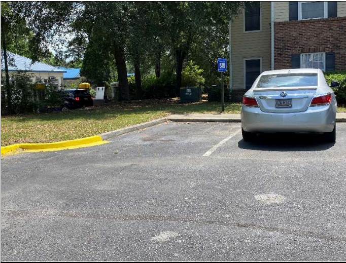
115. Accessible stall without an access aisle, ramp, nor signage
