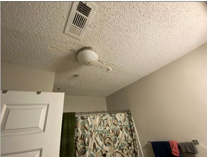
57. Stained ceiling in unit H102 due to active/former plumbing leak
