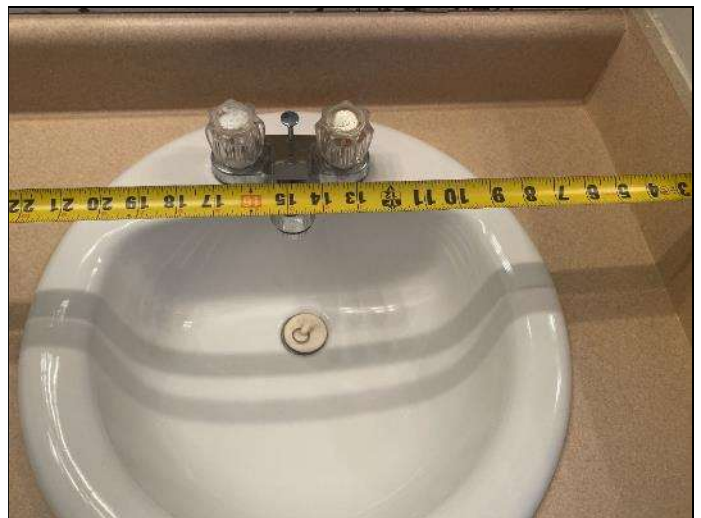
120. 3 BR master bathroom without a lavatory clear floor space
