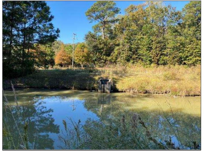
14. Retention pond; note tilted standpipe
