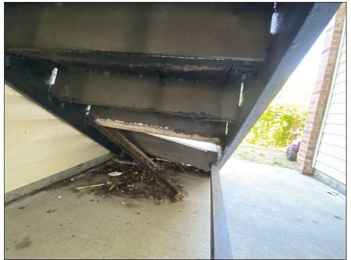
64. Corroded riser at a first flight of stairs
