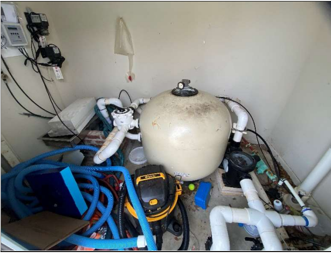
37. Pool pumps and filter
