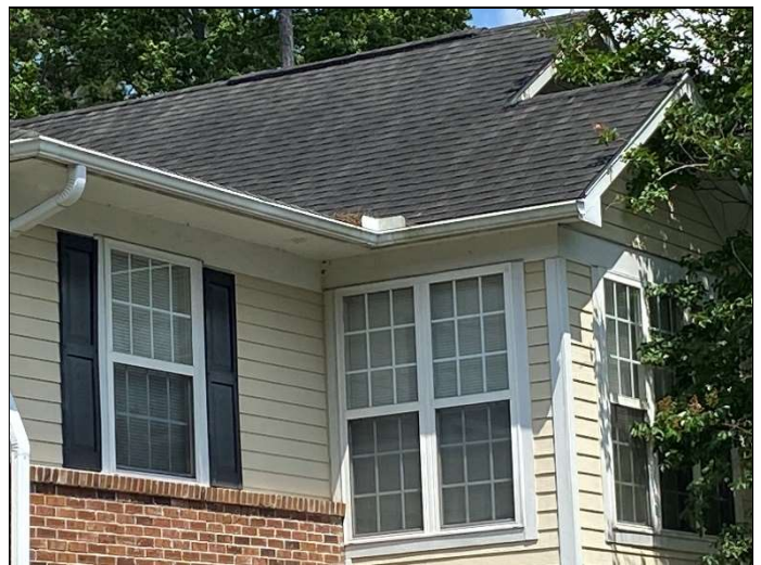
60. Gutters clogged with debris
