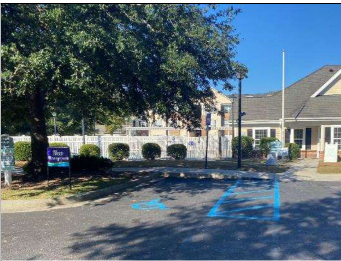
113. Office van accessible stall with noncompliant aisle width and ramp access
