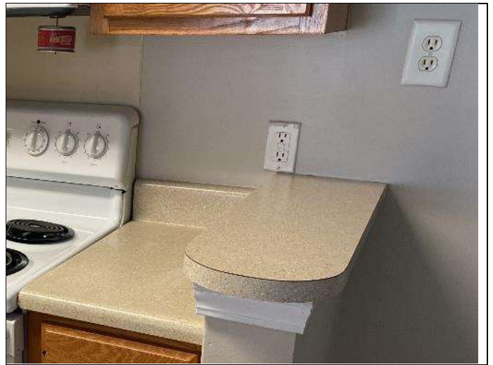
76. GFCI receptacle protection kitchen outlets
