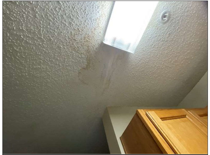
56. Stained ceiling and wall in unit H201 due to active/former roof leak
