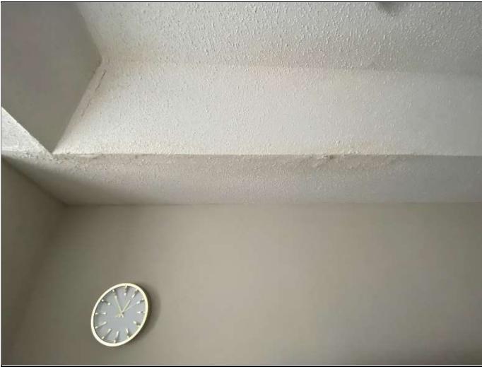
55. Stained ceiling in unit C307 due to active/former roof leak
