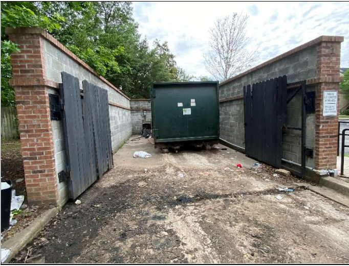
25. Trash compactor. Note: Damaged compactor gate.
