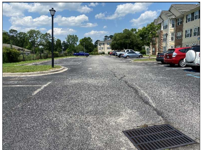
18. Asphalt pavement near Building D; note map cracking
