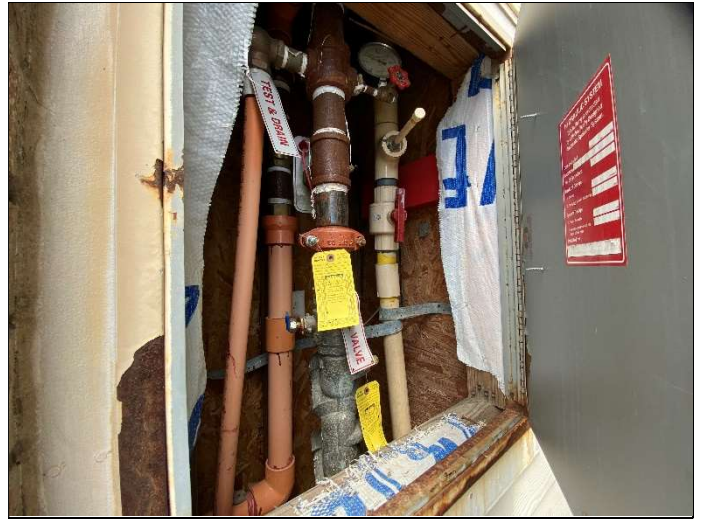
80. Wet-pipe fire sprinkler riser
