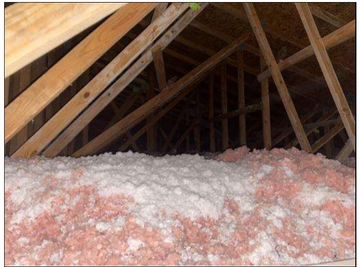
46. Blown-in attic insulation
