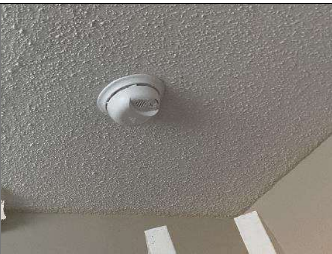
83. Hardwired smoke detector
