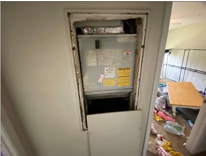
69. Air handler and electric furnace
