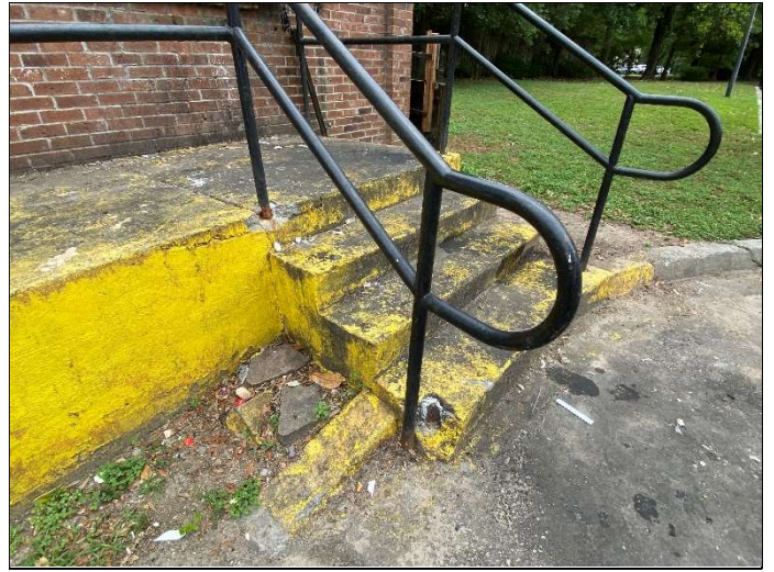
26. Reattach compactor stair railing
