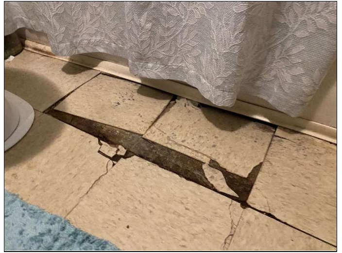
104. Bathroom with VCT flooring. Unit 307 leaking.
